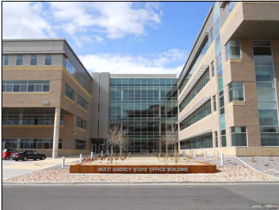
The new Multi-Agency State Office Building on 1950 West.
