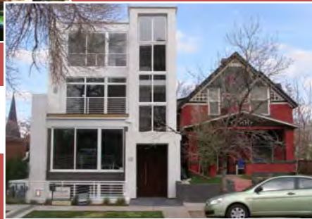
A duplex next to a single-family dwelling
