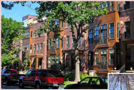
Multi-level attached single-family dwellings
