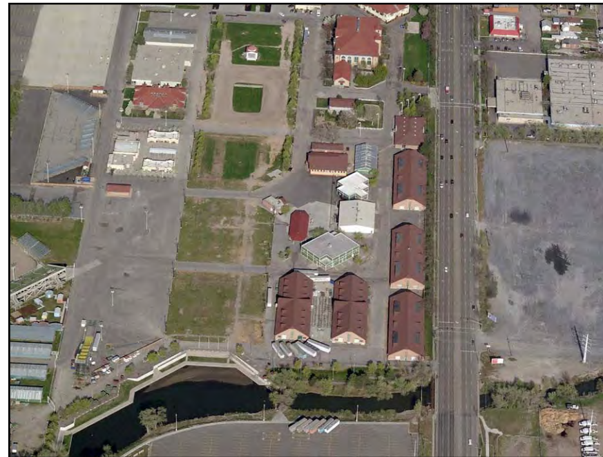
The Utah State Fairpark and the Jordan River looking to the east from the air.
